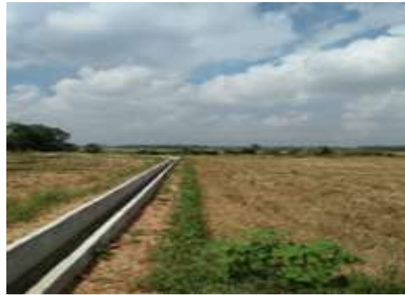
Figure 15: Canal constructed by the project in Medirigiriya
