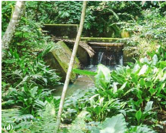
Figure 3: (a) Hilly areas of the Nilwala downstream and (b) small tributaries, (c) water springs and (d) anicut systems
