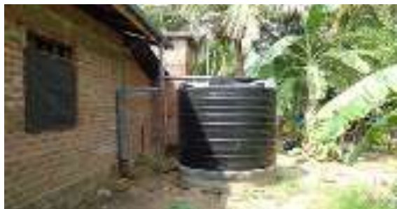
Figure 10: Rainwater harvesting tank
