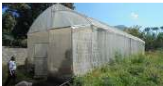
Figure 13: Standard polytunnel built by the project
