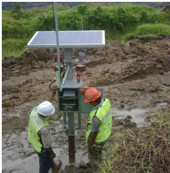
Figure 7: EW system being installed by NBRO
